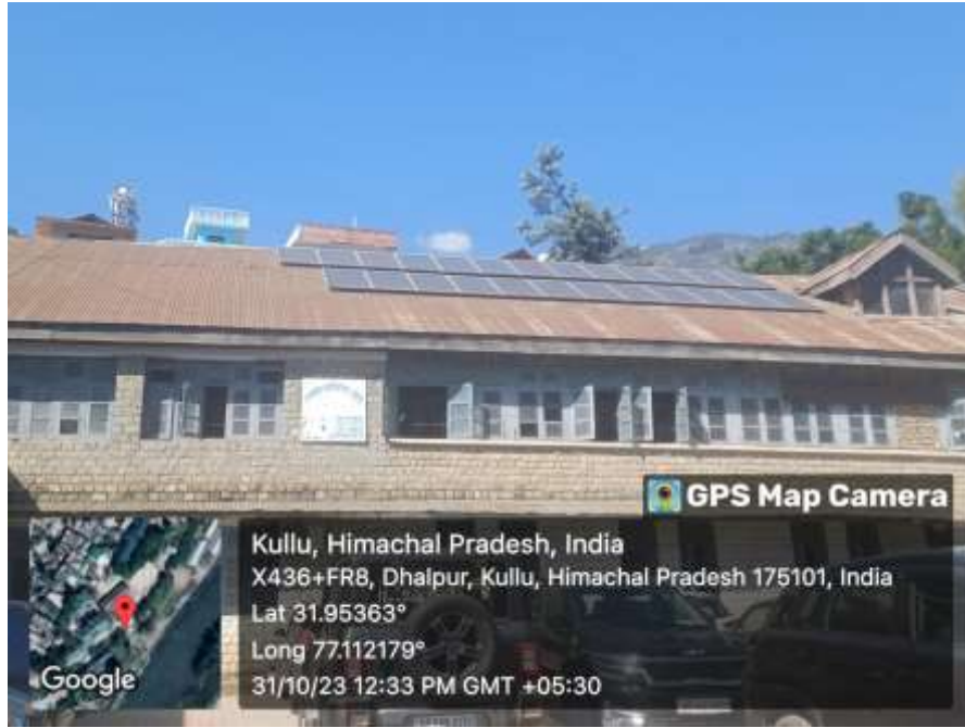
Figure 3: Solar Plant at Library & Science Block (11 kWp)
